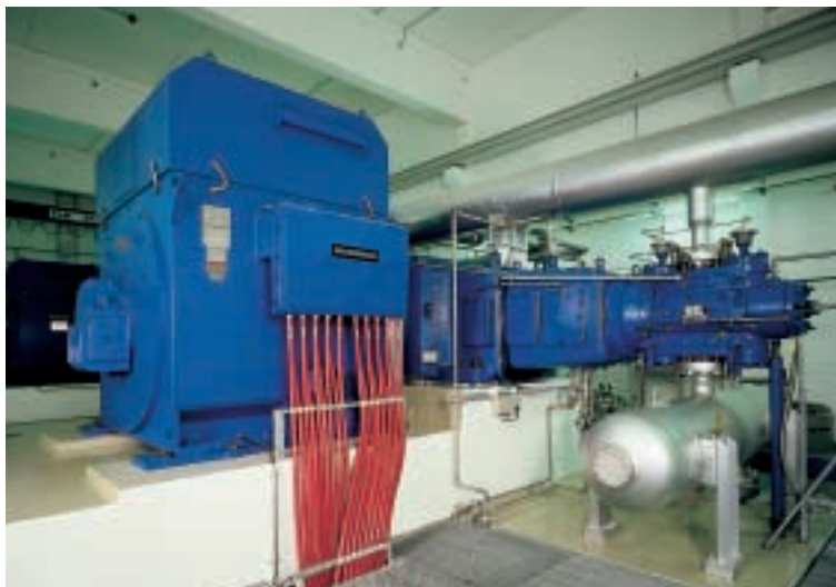
Piston-type gas compressor, driven by a converter-fed motor, 1,900 kW, 2 x 920 V, 14 poles, IP55 with top-mounted water/air heat exchanger IM B3
