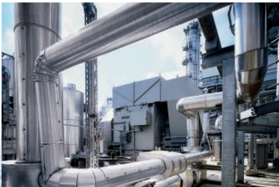
Piston-type gas compressor in an oil refinery, 3,500 kW, 6 kV, 18 poles, non sparking Ex nA II, IP55 with top mounted tube-type air/air heat exchanger, IM 1205
