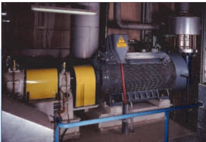
Flue gas fan, driven by a motor 600 kW, 6.3 kV
