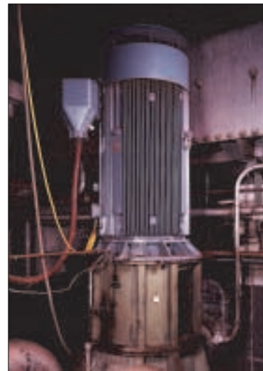
Condensate pump, driven by a motor 800 kW, 6 kV
