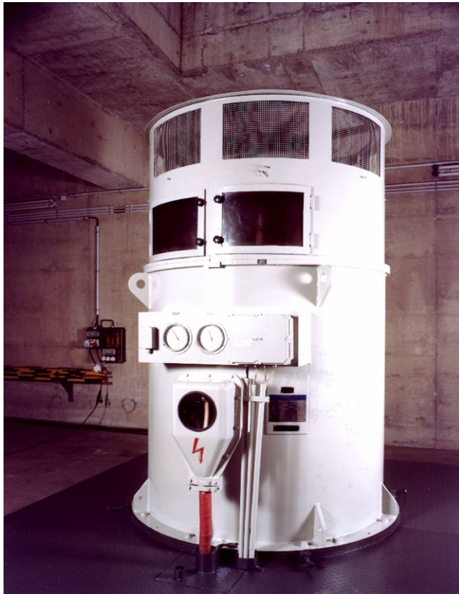
Pump drive, 2,250 kW, 6.3 kV and 1492 rpm
