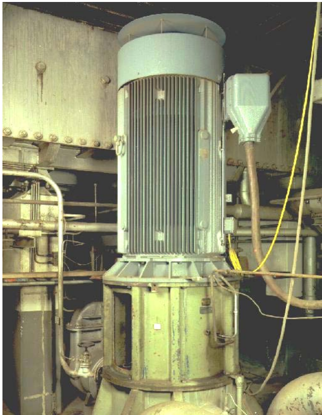
Pump drive, 800 kW, 6 kV 1493 rpm
