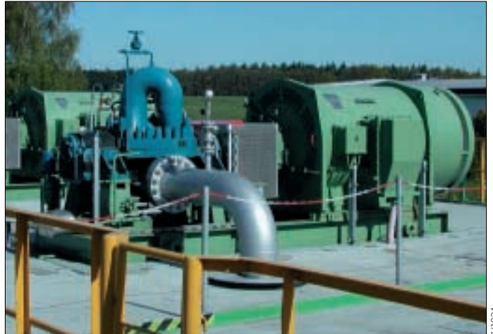
Pump drives in a pipeline booster station, Exd(e) IIB T4, 1,450 kW, 6 kV, 2pole
